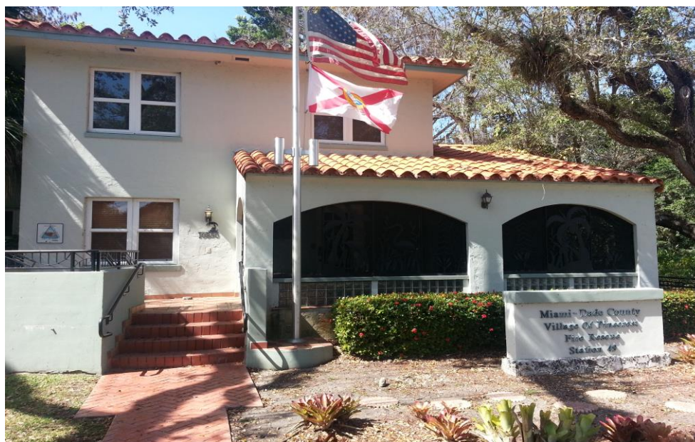
Figure 3. Miami-Dade Station 49 (Pinecrest), 10850 SW 57 th Avenue
